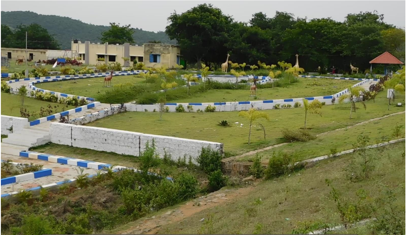
At the entrance of dam: A large park and buildings for staff to stay
