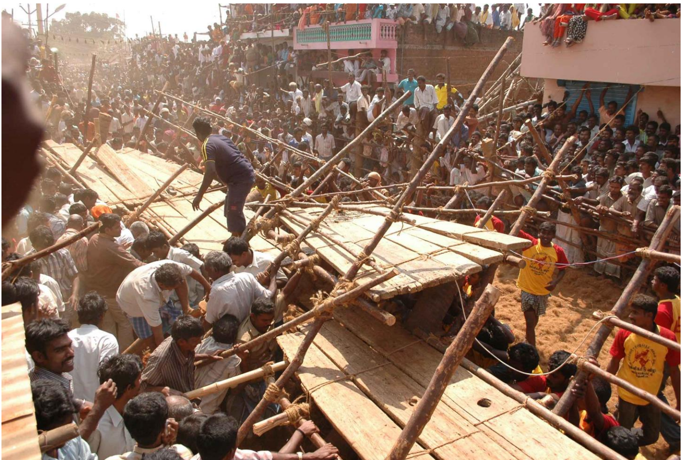
Unsafe gallery collapsed leading to serious injuries
